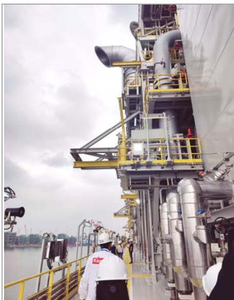
VIEW OF ONE OF FOUR LNG PROCESSING TRAINS ON THE VESSEL
